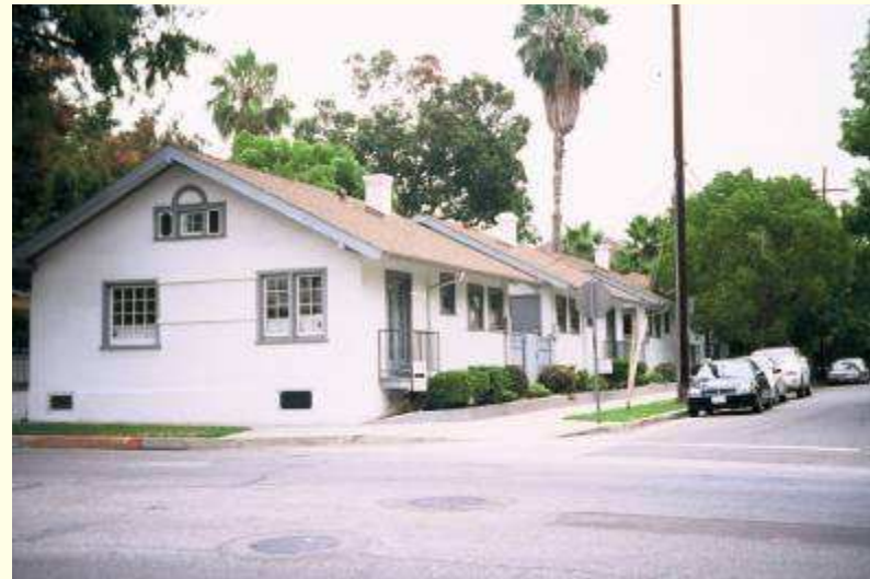
PASADENA COURTYARD HOUSING
