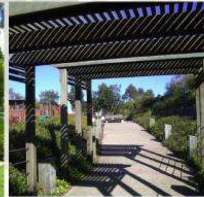
Shade structures provide comfort for journeys
