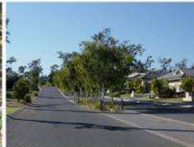
Central drainage swale in road corridor
