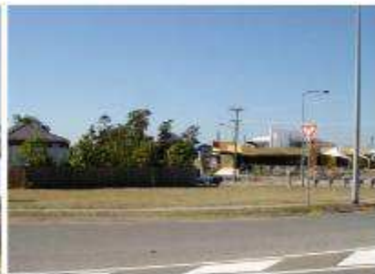
Poor relationship between residential areas and tavern. Back fences of medium density housing line street.
