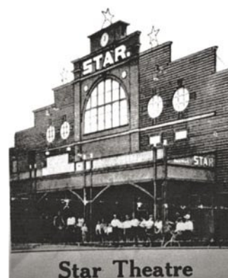
Former Star Theatre, Florence St (Coles site)
