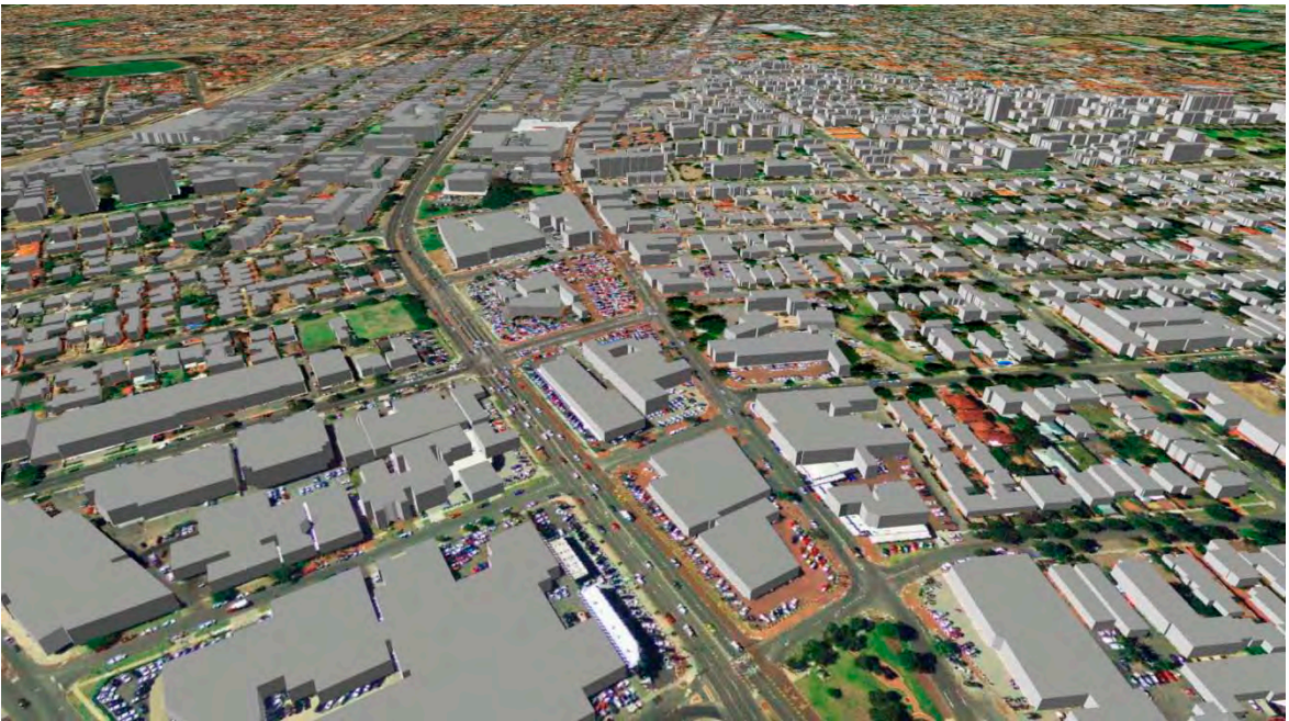
VICTORIA PARK (WEST) – VIEW EAST
