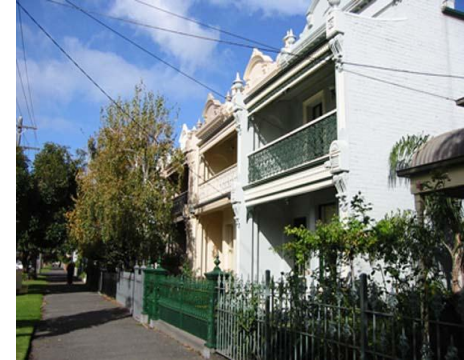
Traditional terrace house
